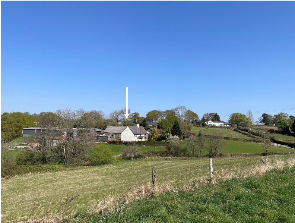
Plate 56: Looking north-east towards Little Creigydd from the west side of the fence line shown below the hillcrest in Plate 55 (the other visible whitewashed property is Yew Tree House)
