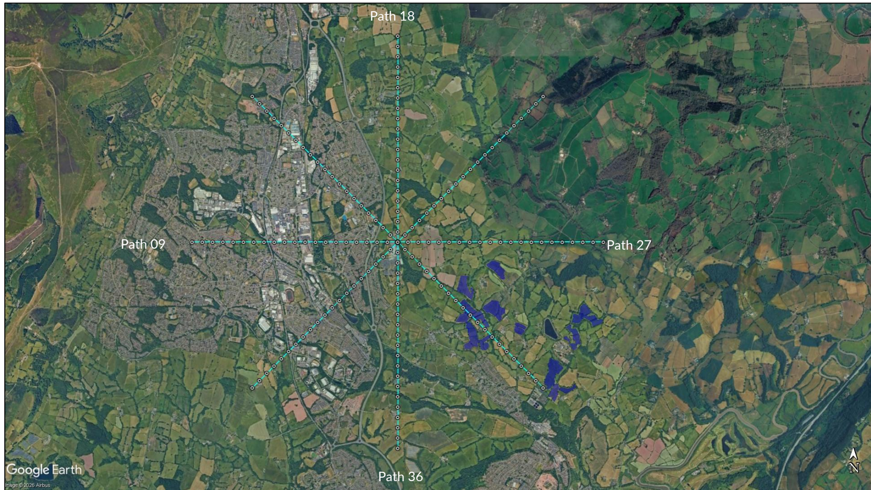
Figure 4 Grange Hospital Heliport approach paths – aerial image
