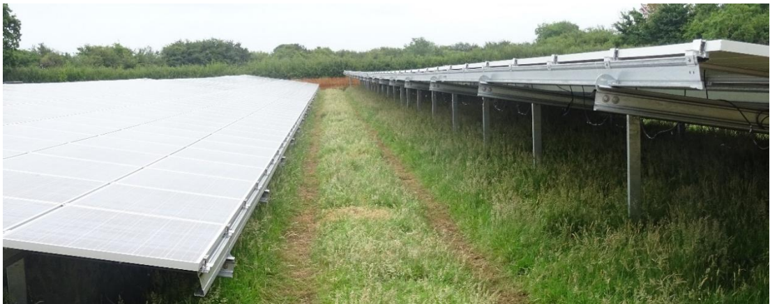
Photo 25: Part installed panels (Bentham Farm, Purton)
