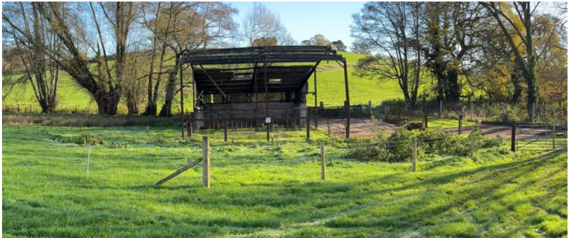
Photo 14: Unused Farm Building, Parcel 8
