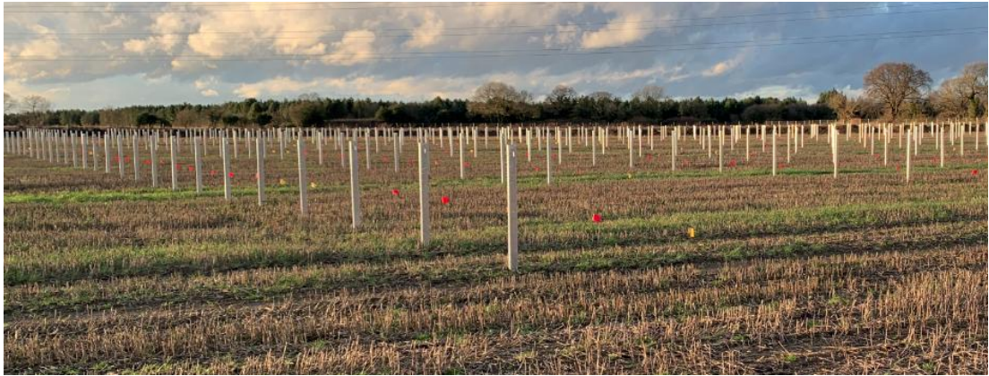
Photo 24: Framework posts being installed (taken at Tiln Farm, Retford, in January 2023)
