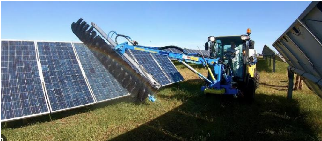
Photo 35: Cleaning of solar modules
