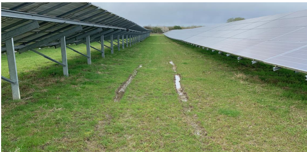
Photo 36: Example of minor ruts caused by vehicles
