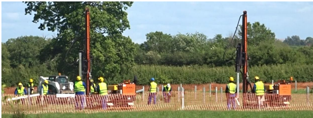
Photo 23: Framework piles being installed
