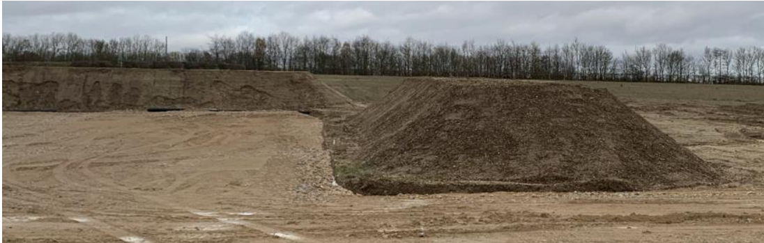
Photo 33: Topsoil Storage Example
