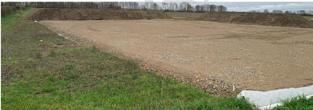
Photo 31: Newly-laid Construction Compound (Elsham-Lincoln Pipeline)
