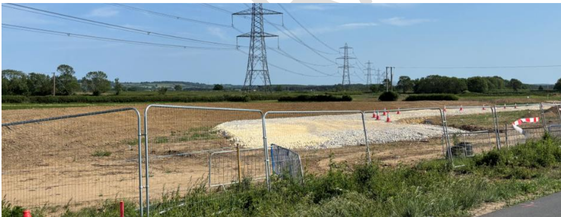
Photo 30: Temporary Site Access (North Hykeham Relief Road)
