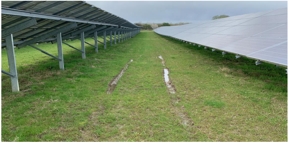
Photo 57: Ruts Caused by Vehicles
