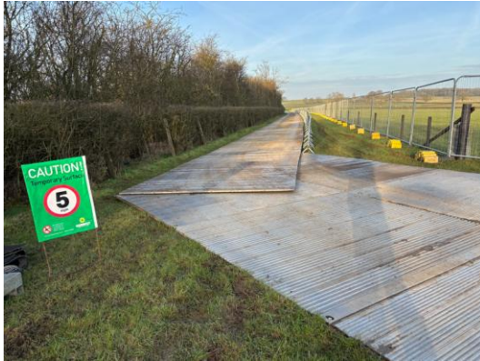
Photos 28 and 29: Temporary Track Construction
