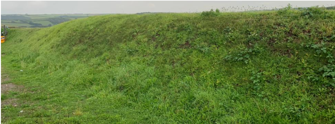
Photo 34: Grass-seeded Soil Storage
