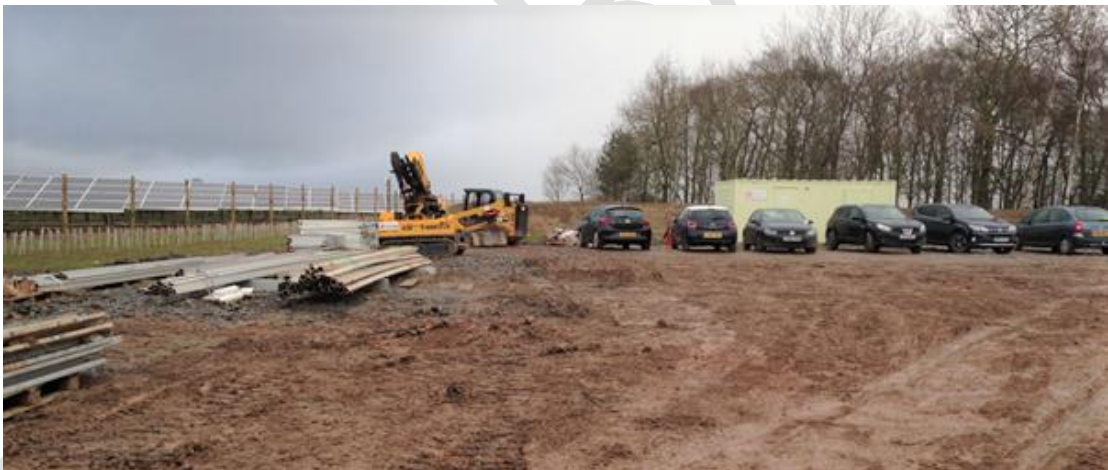
Photo 35: Start of Restoration of Construction Compound
