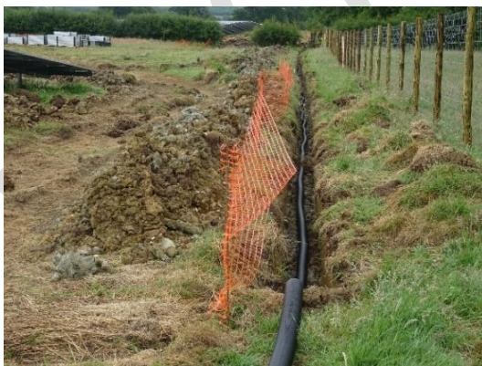
Photos 44 and 45: Cable Installation
