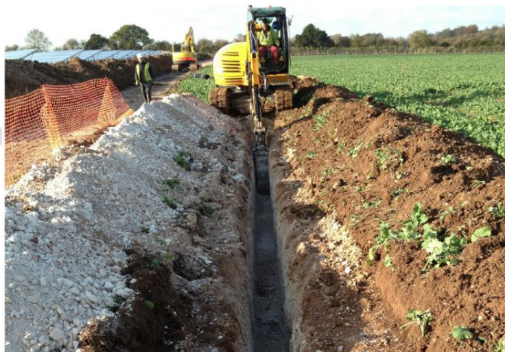
Insert 21: Machinery Used for Trenching
