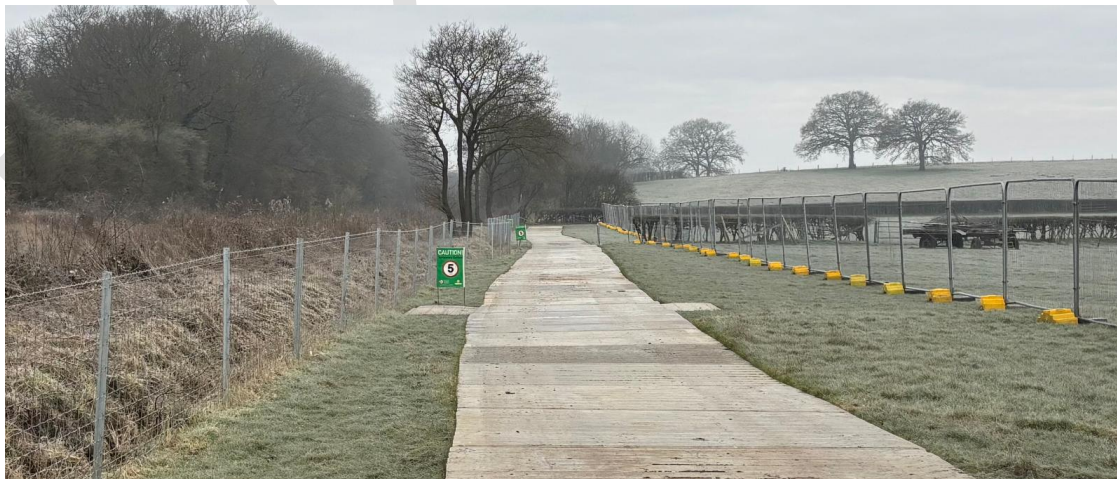
Photo 17: Example of Temporary Matting
