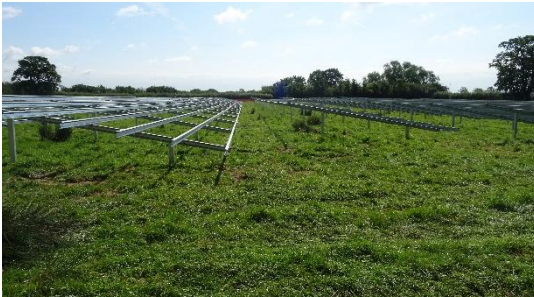
Photos 37 and 38: Ground After Construction
